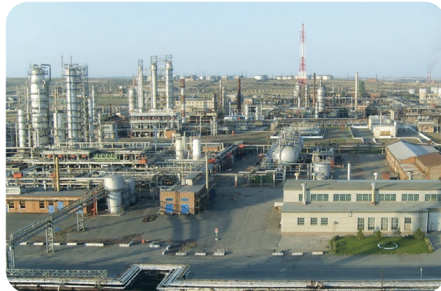
Orsky oil processing plant. Package of firefighting equipment. Customer: Electrosnabsbyt, Orsknefteorgsynthes.
