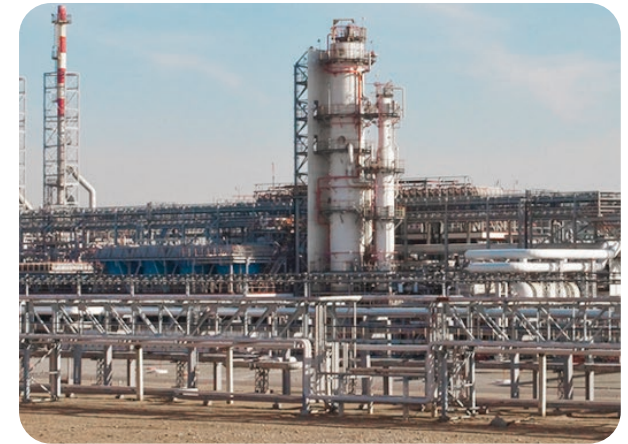
Lukoil-Volgogradneftepererabotka. Block container for fire suppression, firefighting equipment. Customer: IC Technohim
