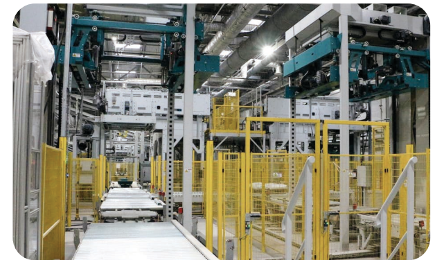
ZapSibNeftekhim (SIBUR). Logistics platform. Firefighting equipment, foam generators, foam concentrate storage and dosing system, foam concentrate Aquafoam. Customer: Yamata Endustriel (branch)
