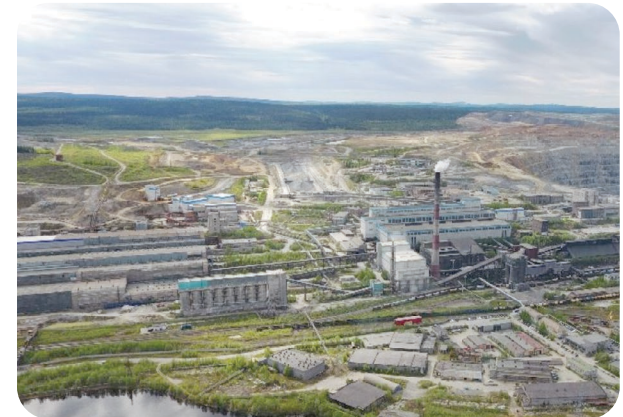
Kovdorsky Mining and Processing Plant. Fire equipment complexes. Customer: AES – Trading House
