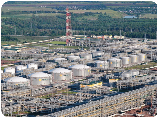
Tank farm in Almet'yevsk. Fire equipment complexes. Customer: TANEKO, TATNEFT
